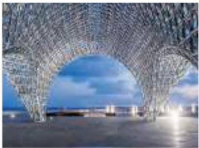
Heavy Steel Structure
